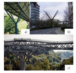
Figure 9. Germany bridge structural designs inspired by trees: a) Nsnback St. Bridge, Germany (Structurae, 2002);b) Hserning St. Bridge, Germany (Structurae.net); c) Tabiat Bridge, Iran (Guideiran, n.d.)
