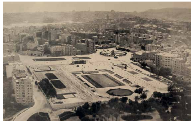
Fig. 3. Taksim Square and the İnönü Promenade (Gezi Park) c. 1940s. (Reproduced from Güzelleşen İstanbul , Istanbul Municipality, 1943)
