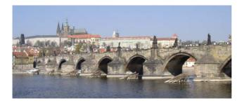
**Fig 1.** Charles Bridge with 16 arches and a clear span of 16,62 m to 23,38. The overall bridge length is 515,76 m and it is 9,4 m wide. The dimensions of massive stone piers at the arch footing range between 8,5 m and 10,84 m by 24,0 m to 25,0 m. Pier heads have been "sharpened" against the water stream at an angle of  $65^{\circ}$ . The bridge construction started in 1357 and was completed in 1406
