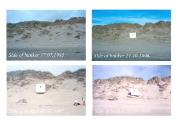
Fig. 3b. View from the south side of the bunker. Observe the exposure of the south-facing window and undercutting of the concrete platform
