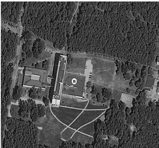
Fig. 3. Latvian rehabilitation centre Jaunkemeri. The Situation aerophoto, Jurmala. Source: compiled by Balode (according to literature review based on (Google... 2014))
