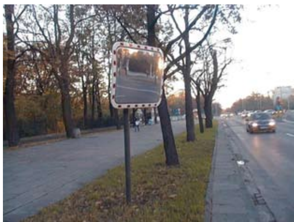
Fig. 7. View of mirror placement on the road with the lack of visibility
