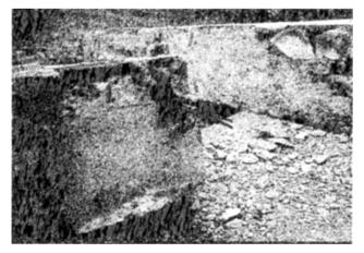
Fig 12. Rupture of bridge staircases due to corrosion of prestressed tendons
