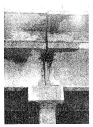
Fig 9. Deterioration of edges of beams and cap of pier due to leakage of expansion joint
