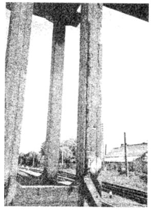
Fig 4. Corrosion of reinforcement of the multiple-column pier accompanied by cracking and deterioration of concrete cover
