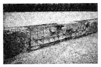
Fig 8. Detail of damaged reinforced concrete parapet in the splash zone
