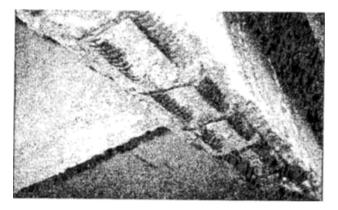
Fig 5. Debounding and corrosion of longitudinal bars and stirrups of reinforced concrete bridge beam
